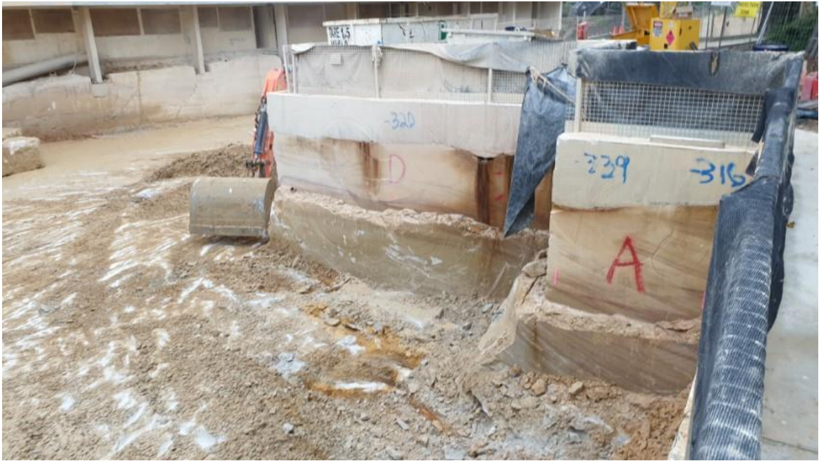
Image 23: Bulk excavation to the northwest end of the site.
