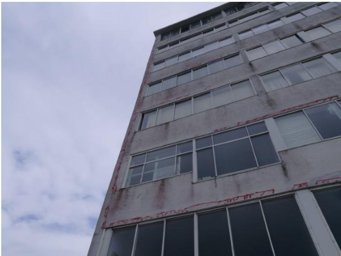
Image 10: Red markings on southeast facade indicate locations of drummy concrete due to the underlying issue of concrete spalling
