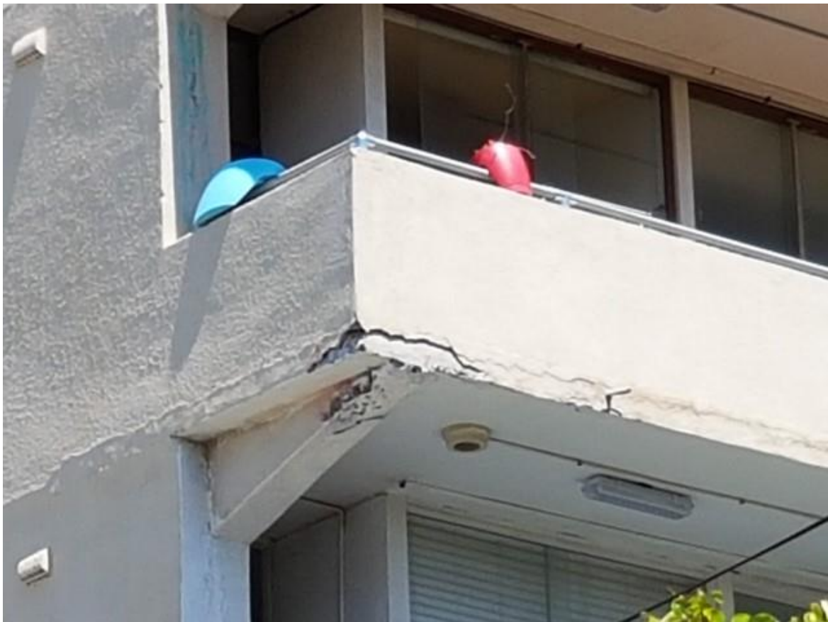
Image 13: Concrete spalling to western walkway
